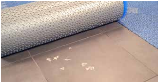
Existing cracked tile
