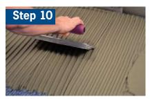
Use the appropriate notched trowel to comb the mortar, then install the tile or stone directly onto the membrane.
