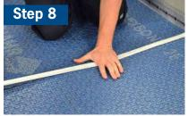
Cover the joints with self-adhesive ARDEX UD 156 Movement Joint Tape to protect against the entry of mortar and grout.
