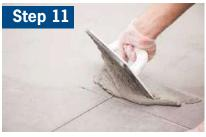
Due to properties of plastic membranes, mortar type, tile type, tile size and climactic conditions, the mortar curing time required prior to grouting may vary. ARDEX mortars allowable for use with ARDEX uncoupling membranes typically permit grouting in 3 - 24 hours.
