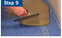
Using the flat side of a trowel, fill and smooth ARDEX UI 720 FLEXBONE with the appropriate ARDEX mortar so that the mortar is flush with the top of the mesh.
