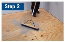
Sweep or vacuum debris from the substrate. In intermittent wet areas or where waterproofing is required, moisture-sensitive substrates, such as gypsum, must be protected from water damage by priming with ARDEX P 51 and installing ARDEX 8+9.
