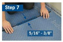
Leave a joint minimum width of 5/16" - 3/8" (8 - 10 mm) for expansion and field perimeter joints that sub-divide large areas, doorways, etc.
