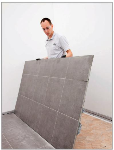
If exchanging the floor covering is desired, spread a polyethylene sheet over the substrate prior to installing ARDEX UI 720 FLEXBONE. The sheet acts as a separating layer between the substrate and the membrane to protect against adhesion from any mortar used during the floor covering installation.
