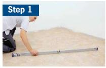
Check the substrate for load-bearing qualities, evenness and structural soundness. If leveling is necessary, a product such as ARDEX Liquid BackerBoard may be used.
