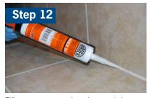
Fill movement and perimeter joints with an appropriate soft joint filler such as ARDEX CA 20 P or ARDEX SX.
