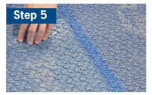
Butt joint the membrane sections with the protruding edges of the self-adhesive mesh weave. Overlap onto the adjacent membranes.
