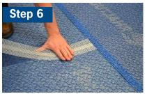
Use the self-adhesive ARDEX UD 158 Seam Reinforcement Mesh Strip to bond seams at the ends and cut areas of the membrane where there is no overlapping self-adhesive mesh.
